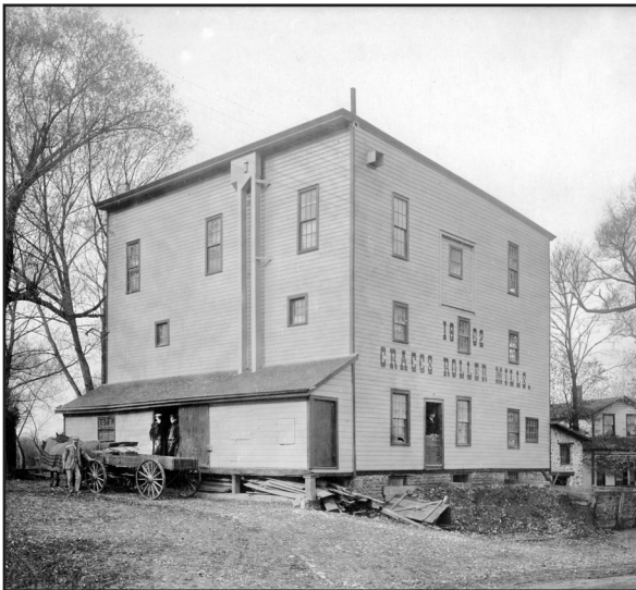
Craggs Roller Mill: prior to 1930 fire
