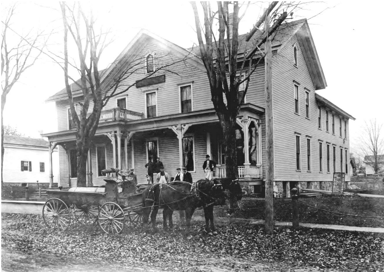
The Pacific Hotel over 100 years ago (top) / and now under renovation (bottom)
