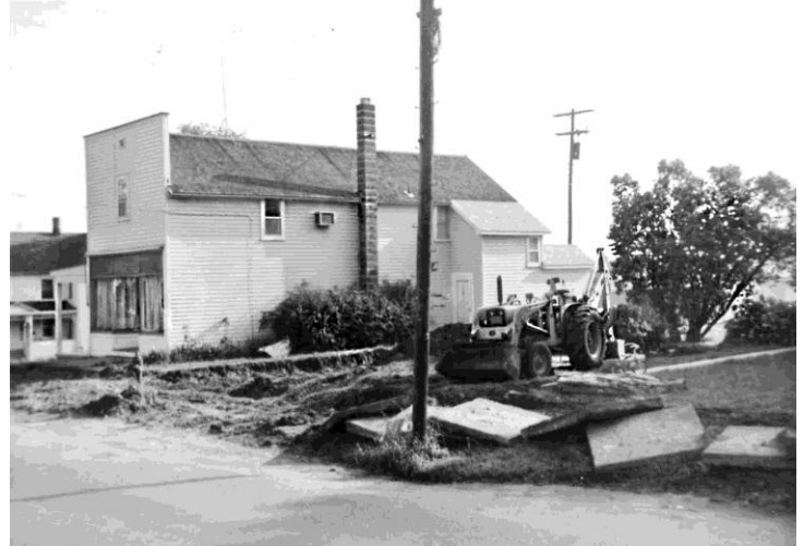
1967: Parking lot installation
