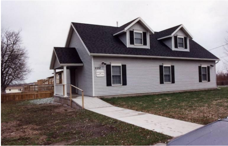
Our museum soon after construction (1989)
