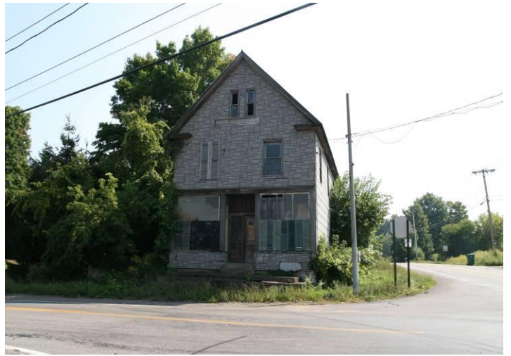
White's store before the 2009 demolition
