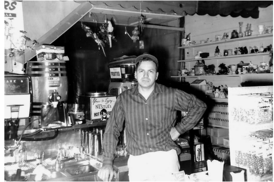
1965: Gordon supervising the remodeling project.
