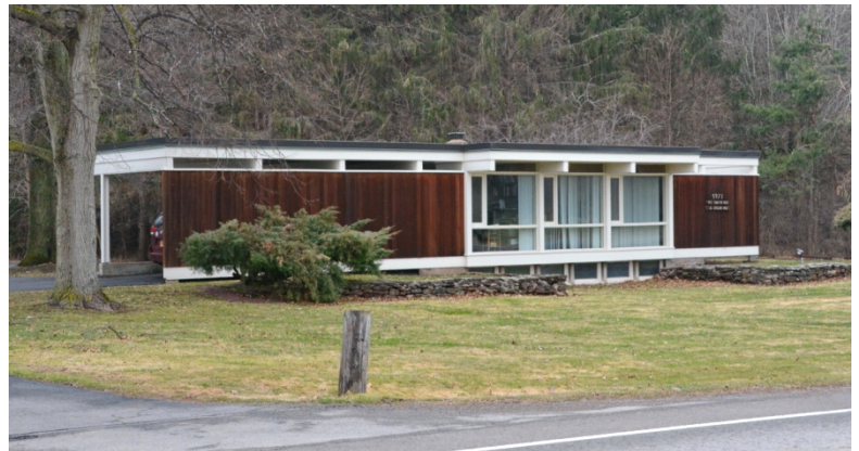
In 1958 Dr. Loomis moved his office to this building on Walworth-Ontario Road in Ontario.
