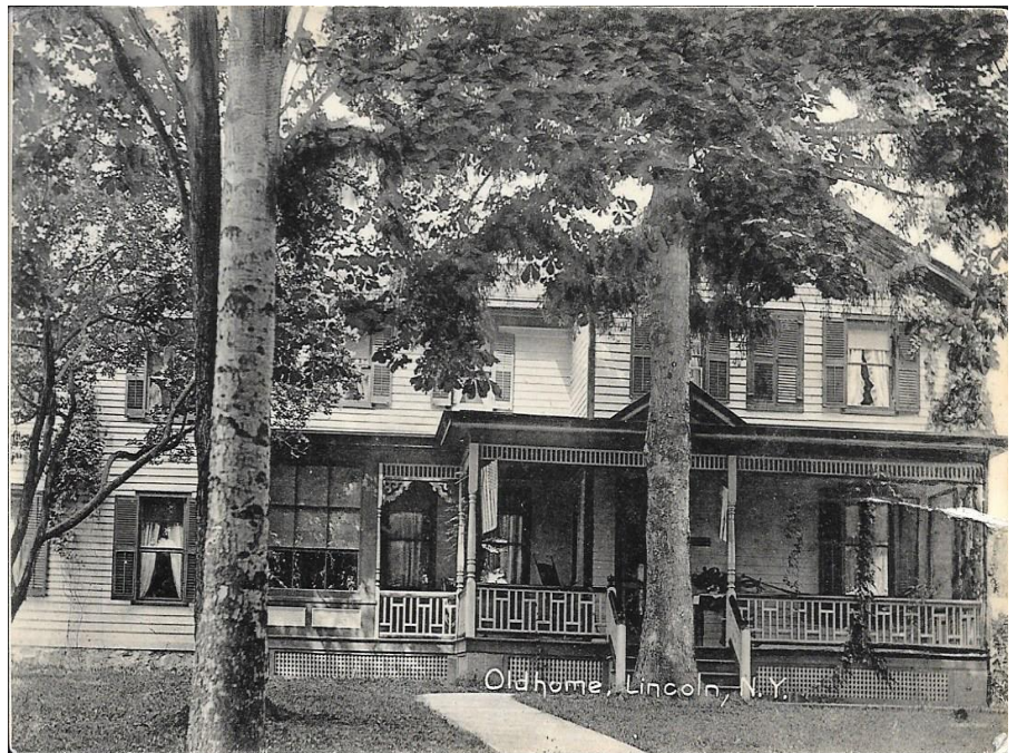
Undated photo of the Peacock/Morris home at 4893 Lincoln Road, now owned by Anita Amsler.
