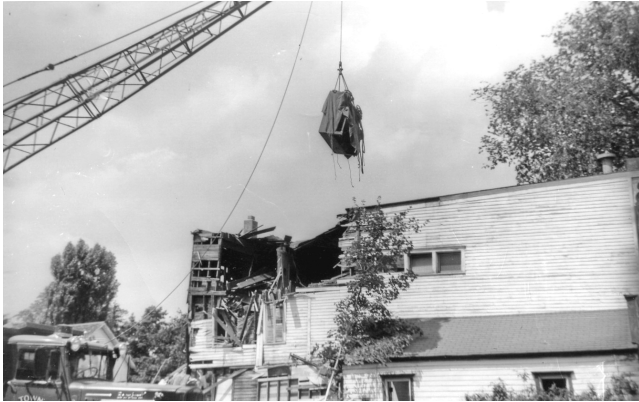
Piano being removed from 2 nd floor meeting room
