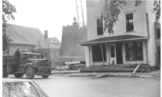
Demolition of Masonic Lodge
