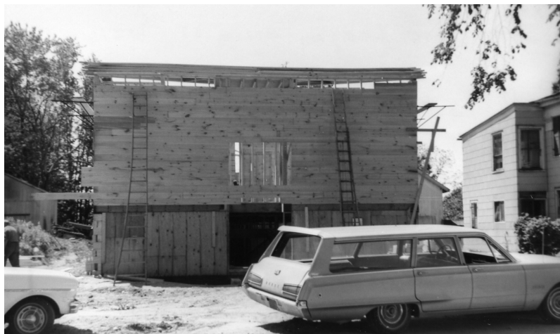
1969: Construction of New Masonic Lodge Above photo courtesy of Gordon Youngman
