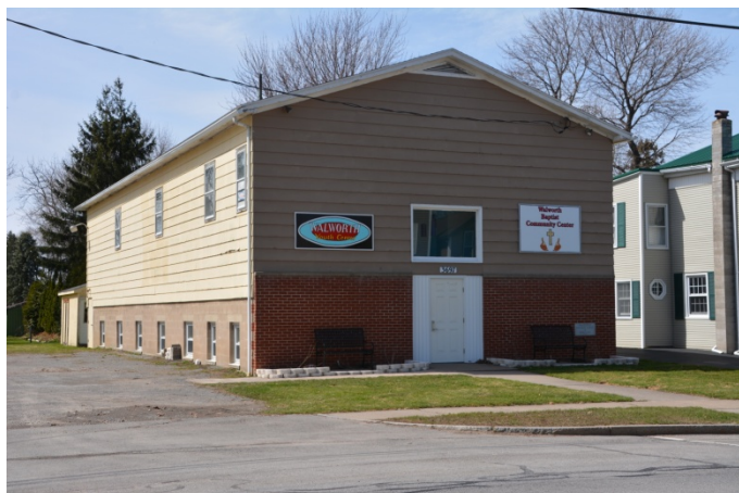
2016 Photo: Walworth Youth Center and Baptist Community Center
