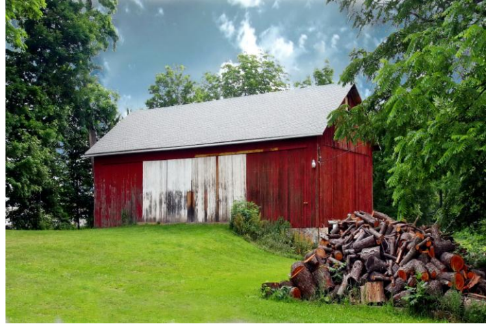
Walworth-Ontario Road barn
