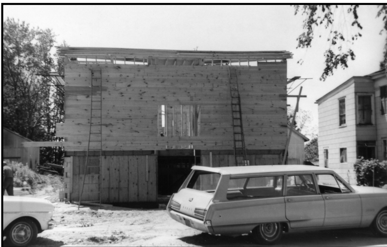
1969: Construction of New Masonic Lodge
