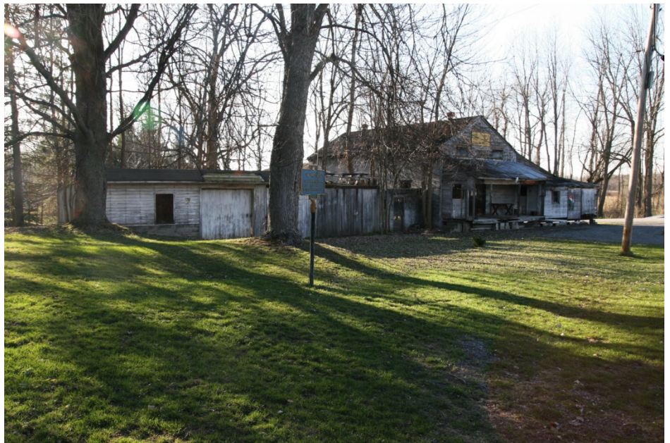
Photo of the old mill at the Huddle (April 2008)
