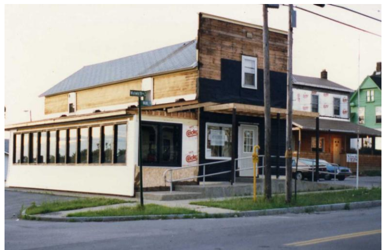
Building the Walworth Laundromat 1987
